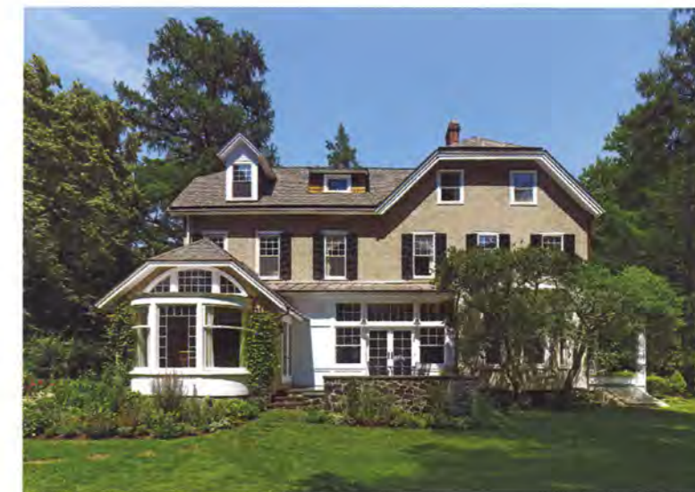
The rear of the house before the renovation (top)—a flat, characterless facade that wasn’t meant to be seen. The rear of the house after the addition of a small projection with a “jerkinhead” roof (bottom). (Courtesy of Voith & Mactavish Architects LLP.)
